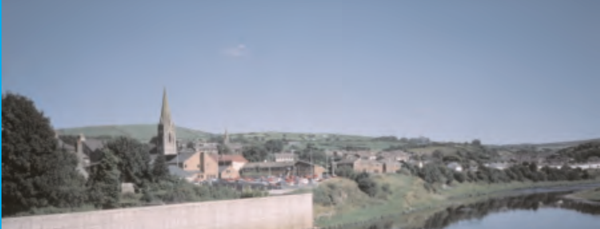
View of flood defence wall
