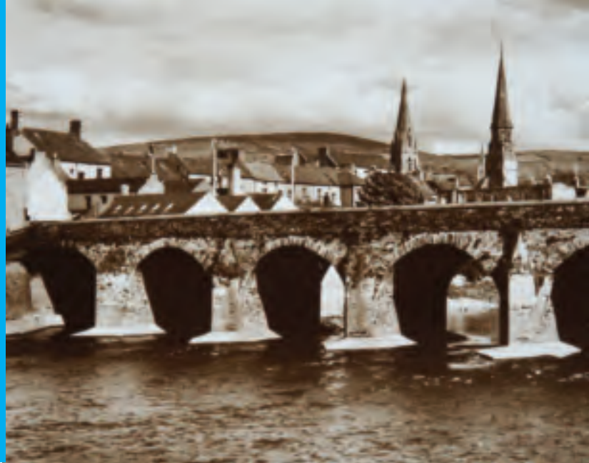
Strabane bridge, viewed from the McGirr area, showing the spires of First Presbyterian Church and Church of the Immaculate Conception.
