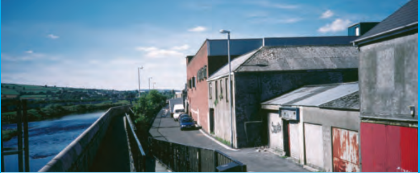
Proposed location for new bridge
