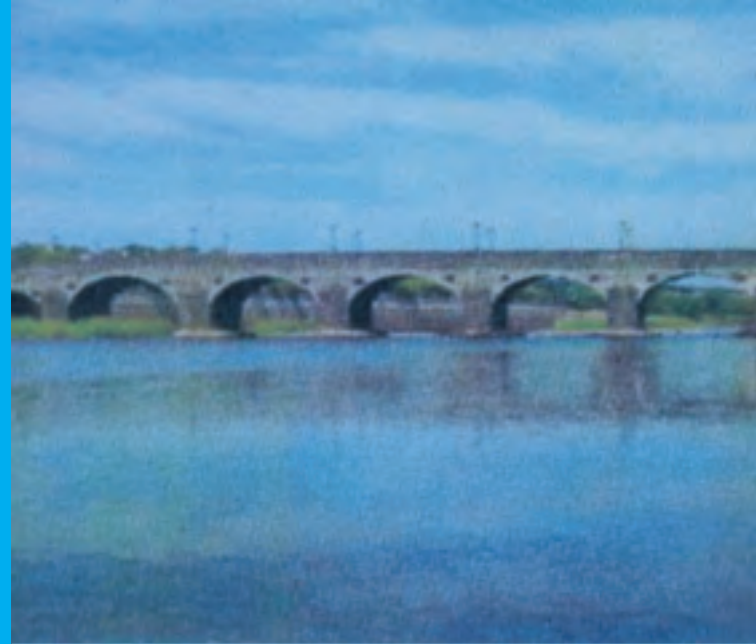
Strabane Bridge post 1990, with the high flood walls on both sides of the river and the concrete feet supporting the arches.
