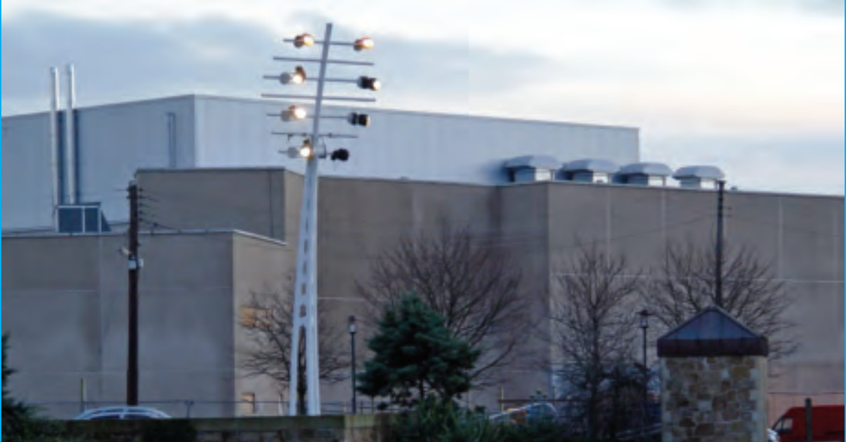
Scene site looking towards Alley arts Centre
